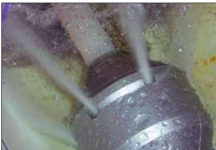
IBAK PHOBOS 1 in operation
