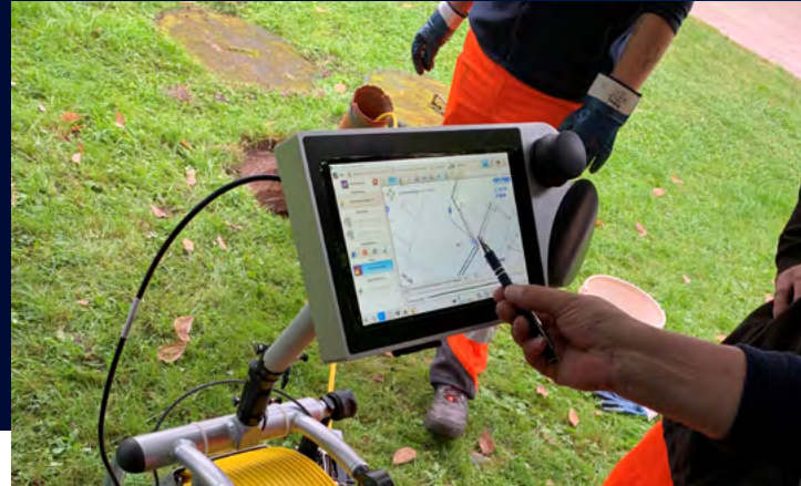
3D GeoSense pipe run surveying with the MiniLite
